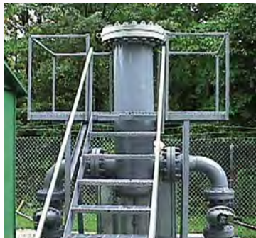
Coalescing filter in service cleaning an eight inch gas pipeline in the midwestern US.
